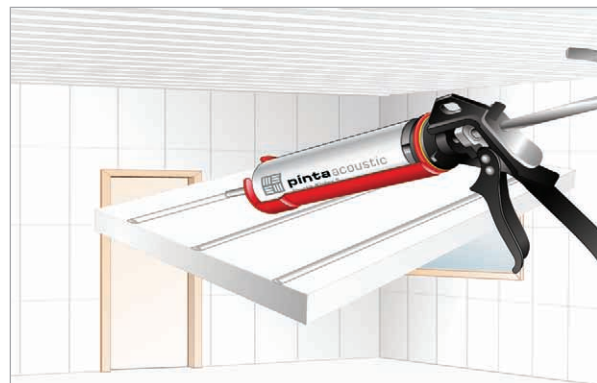
Apply acoustic adhesive
