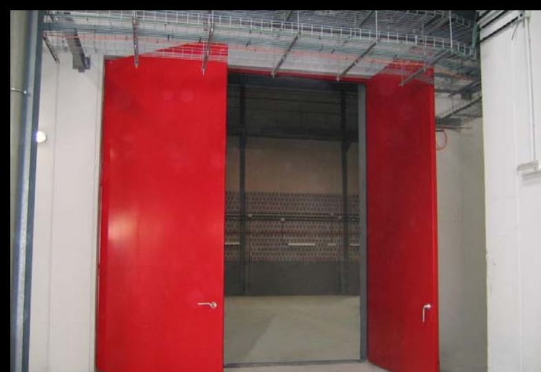
Large dimensions acoustic and fire rated doors
