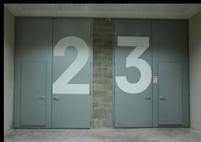
Large dimensions acoustic and fire rated doors
